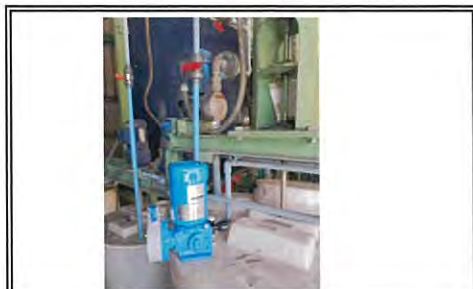
Install chemical pump ( NaOH )
